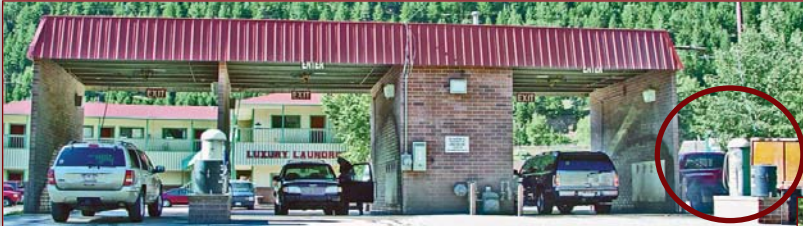
This is a shot of the car wash entrance before the remodel. Circled area shows where the automatic will be built.
